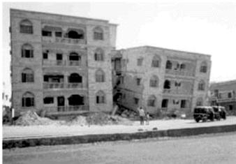
angement. If the builder had constructed according to drawings, he did not follow them. *Two recently constructed five-story buildings collapsed due to soft story effects.*
